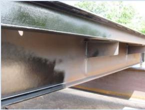
Coal tar undercoat on truck scale
