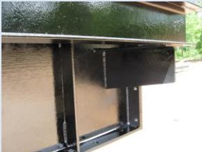
Coal tar undercoat on truck scale
